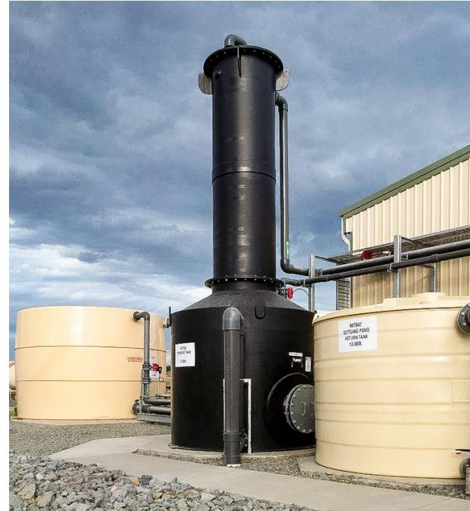
The aim: to fabricate a tower out of high density polyethylene (PE) which would enable the client to remove carbon from the water. This water would already pass through a reverse osmosis (RO) process and, after removing the carbon, enable it to be used in the processing of nitrates.
